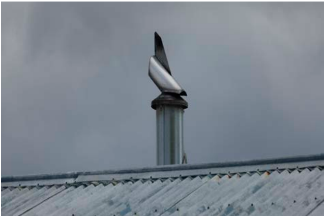
Flue 4 By using the 100-500mm lens at 300mm, the roof, the chimney and flue all give the flue its context, but photographically I don't need the roof or the chimney as the only thing in my mind the flue. This is always the question facing us – how far do we go before we have destroyed our original idea?
