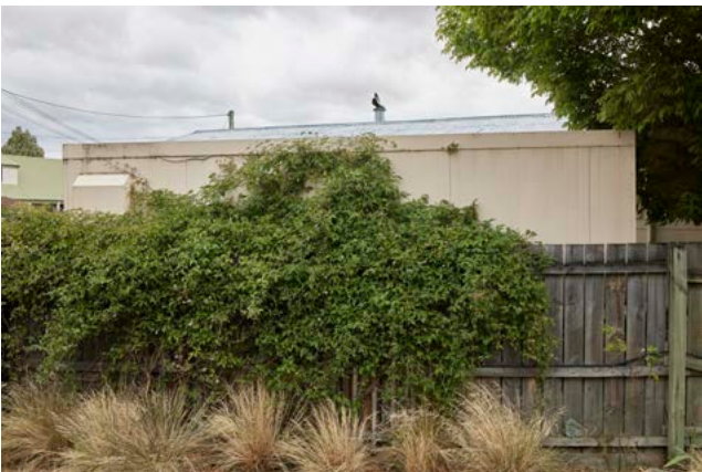
Flue 2 So, I went outside and photographed the flue again, this time at 30mm, but still this framing doesn't tell you what my subject is.
